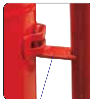
"C" - Hook welded on the cylinder
